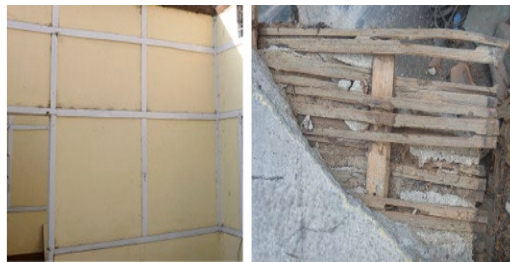
Figure 4. Ekra wall panel. (Dash and Gupta, 2022).
