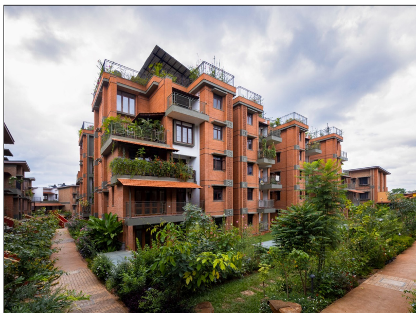
Figure 1 Row houses construction using stabilized mud bricks, Solar PV's and earthen materials at goodearth medley project, Bangalore, India.
