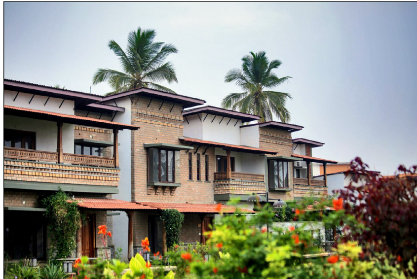
Figure 2 Villa construction using combination of stabilized mud bricks and earthen materials at goodearth malhar project.
