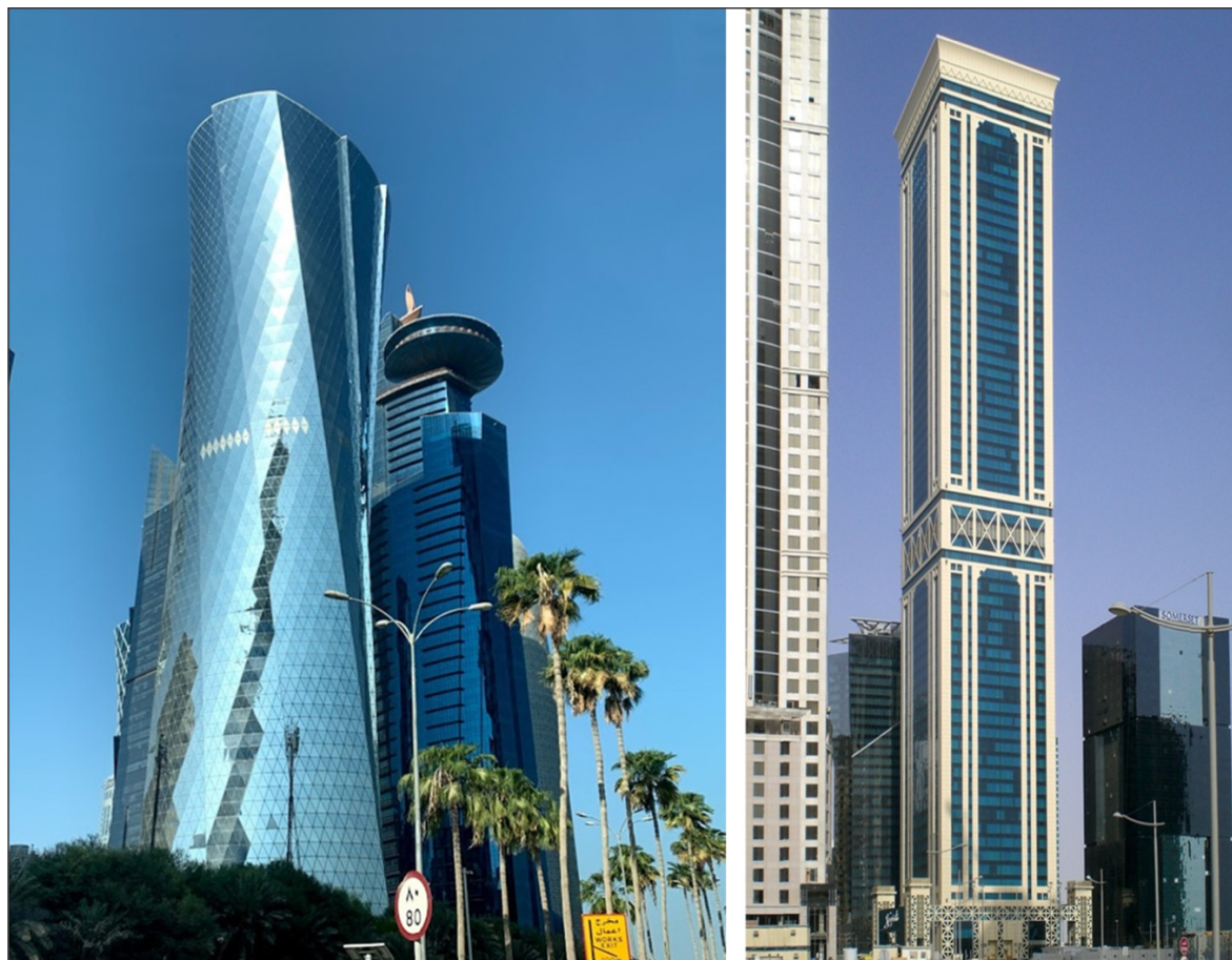
Figure 8–9 Left: Al Bidda Tower and Burj Qatar (Source: Google Earth, 2024), Right: The Kempiski Residence (Suwaidi & Boussaa, 2024).
