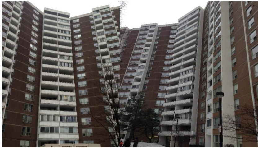
Figure 2. The audited MURB Building (by the author)
