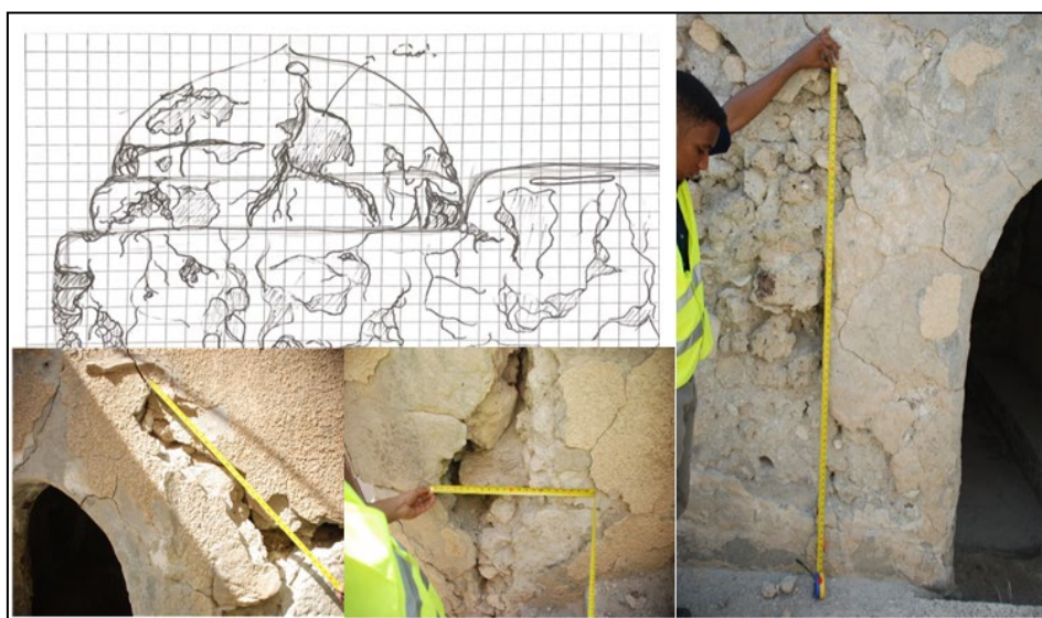
Figure 3. Cracks measurements of Abu Loza's historic bath(Source: Author).
